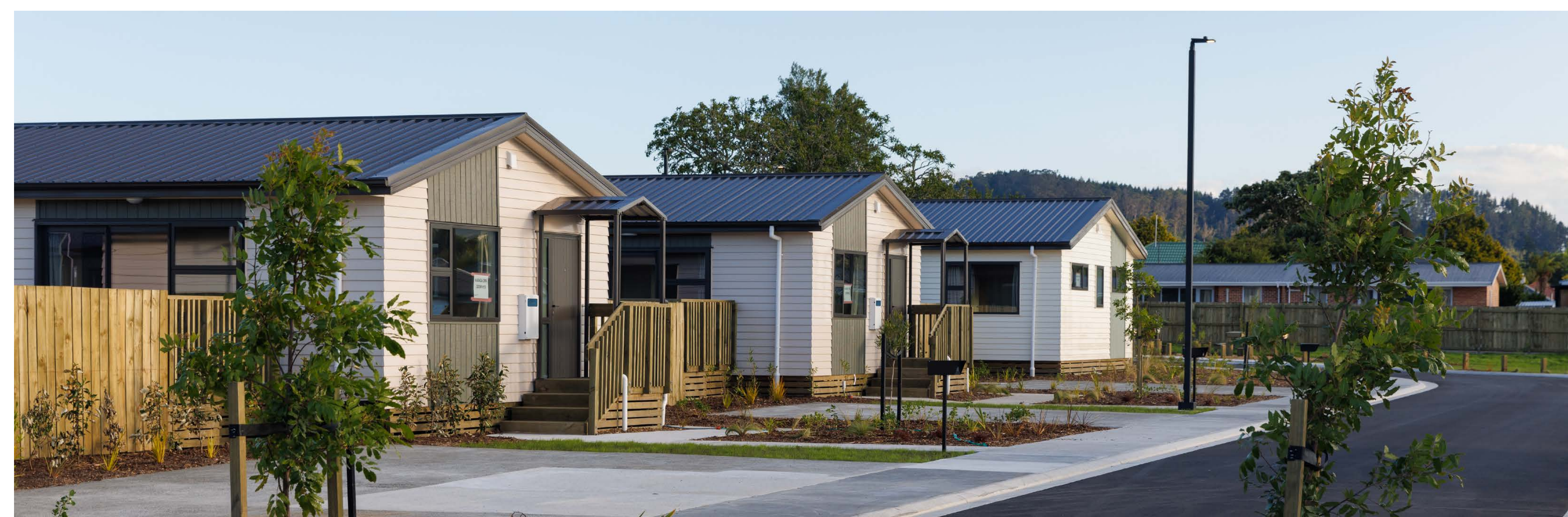
New homes at Ranolf Street / Malfroy Road
