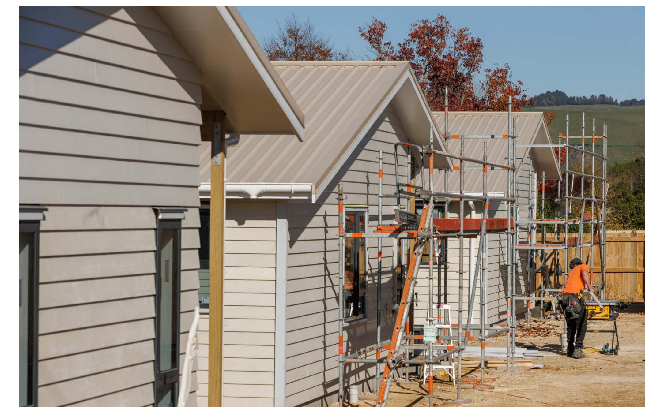
Under construction homes in Rotorua
