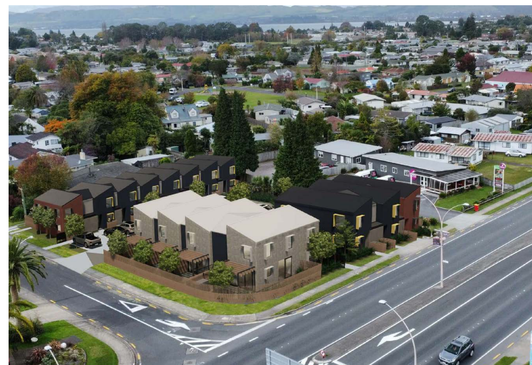
Currently under construction homes at 149-151 Fairy Springs Rd
