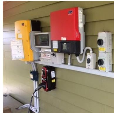
Figure 6 AC and DC disconnects installed next to a wall mounted inverter.
